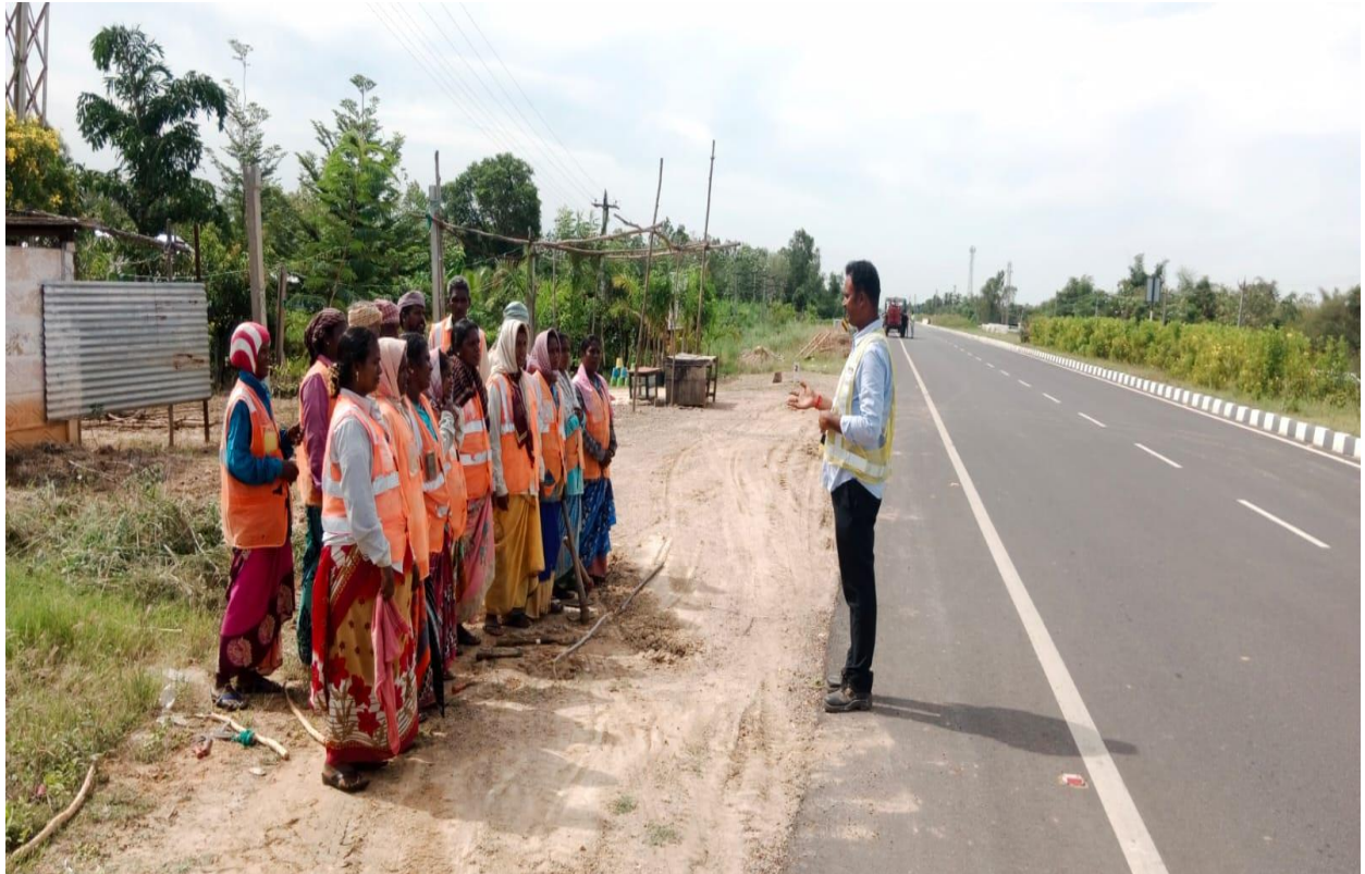
Safety instructions given to labours at Ch. 92+000
